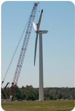
**Figure 2 - 600KW Wind Turbine Installation**
